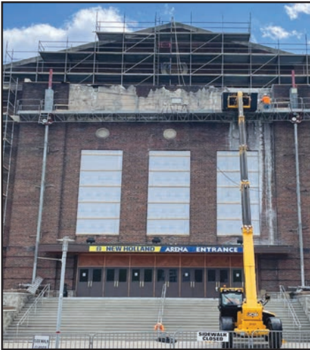
Contractors removing crumbling original panels above arena entrance.
